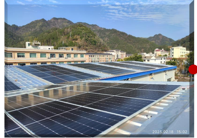
Install Solar Panels
