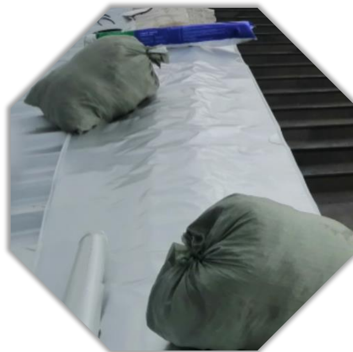
Sealing the Ridge
