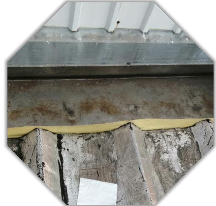
Clean & Dry Surface
