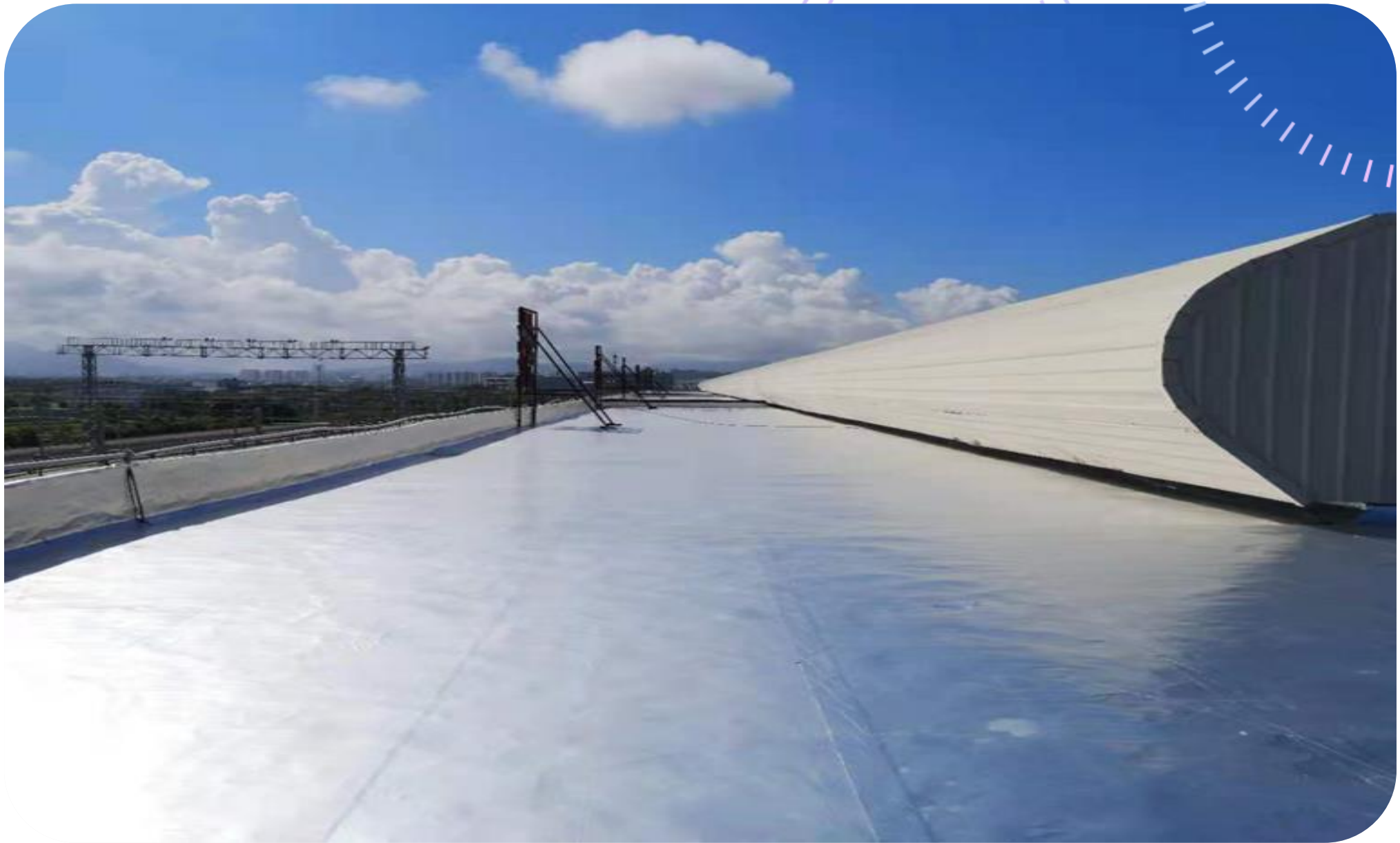
Sanya EMU Station Waterproofing Maintenance China
