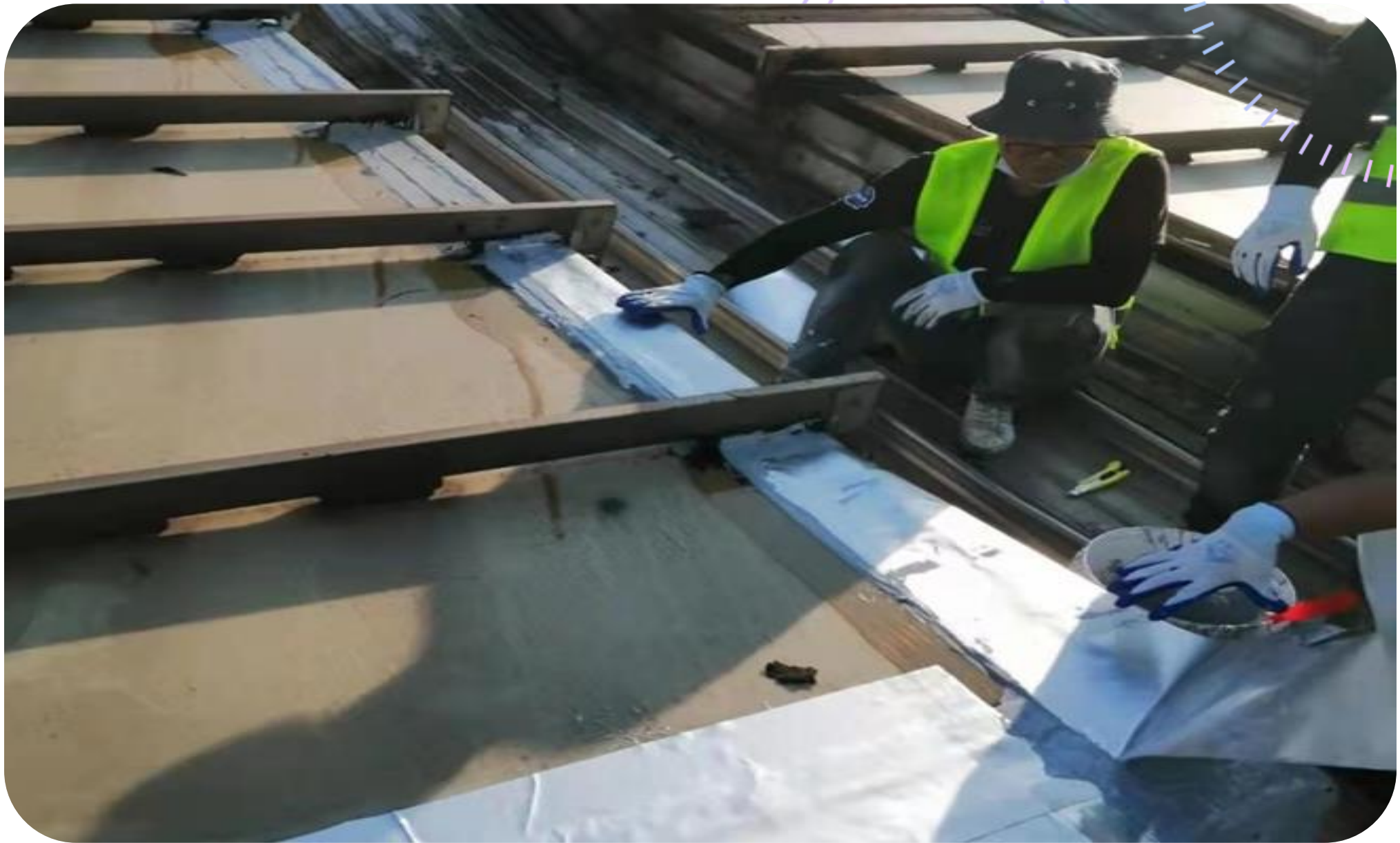
Wuhan Station Waterproofing Maintenance China
